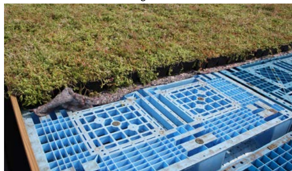
Polderdak in Amsterdam
